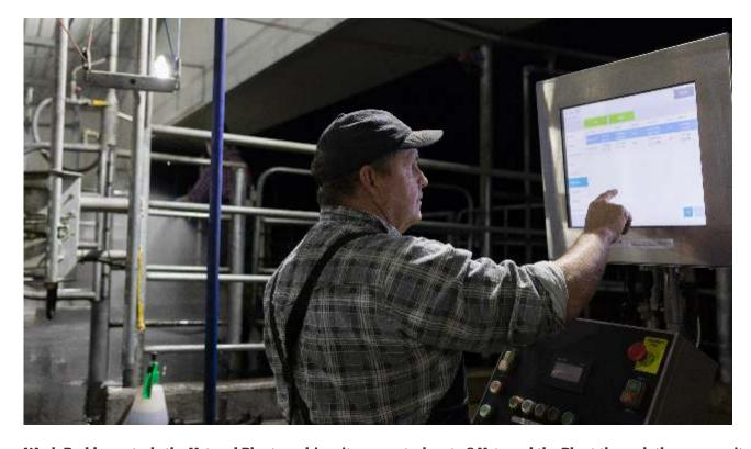
Wash Buddy controls the Vat and Plant washing, it can control up to 2 Vats and the Plant through the same unit.
