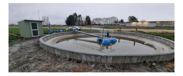
Level Buddy is a system for controlling a pump for either filling or emptying a tank or sump. It uses a submersible level transducer to detect the levels in your tank or sump.
